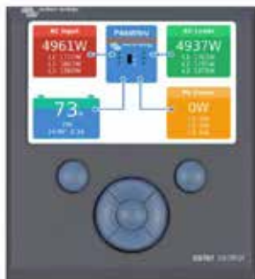
Color Control GX, showing a PV application
